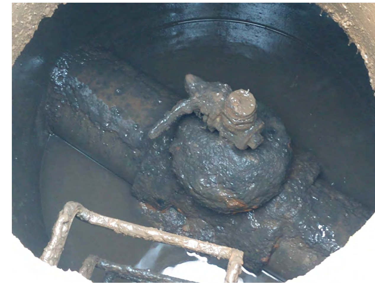
ACCESS POINT-6 INSPECTION PHOTO
