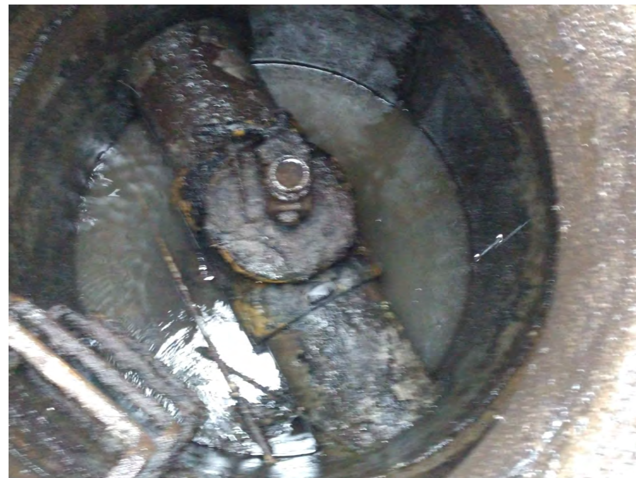
ACCESS POINT-10 INSPECTION PHOTO
