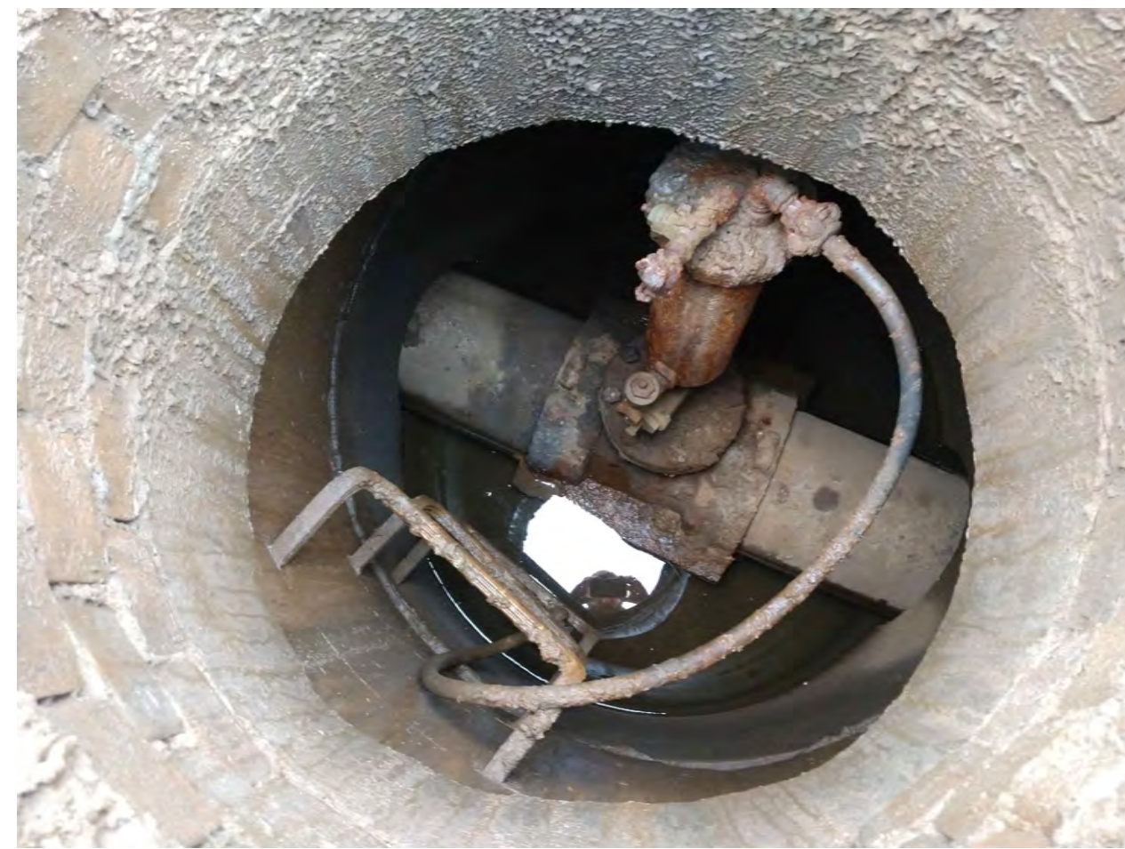
ACCESS POINT-4 INSPECTION PHOTO
