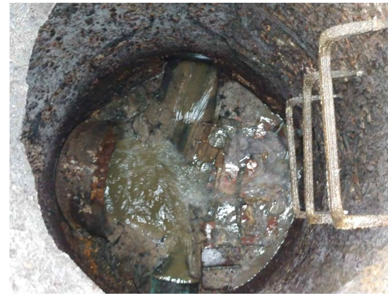
ACCESS POINT-18 INSPECTION PHOTO
