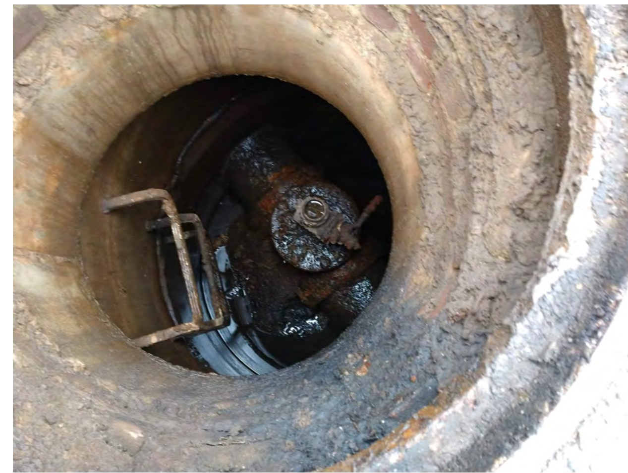
ACCESS POINT-8 INSPECTION PHOTO
