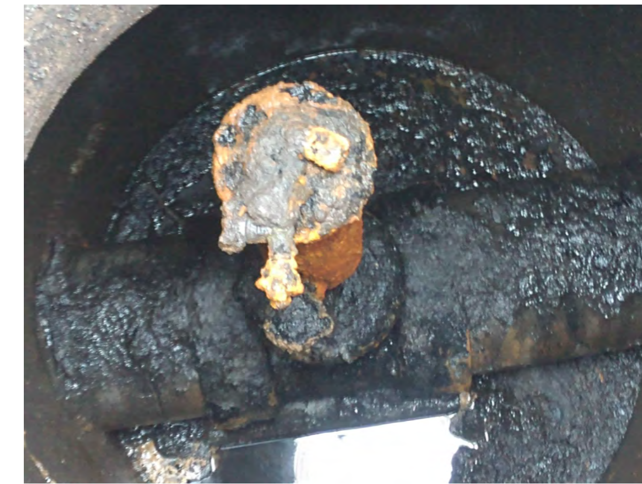
ACCESS POINT-9 INSPECTION PHOTO
