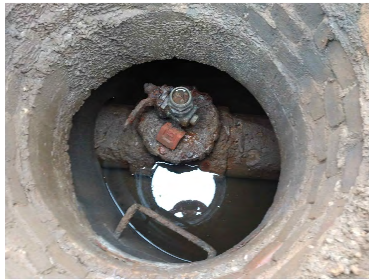
ACCESS POINT-7 INSPECTION PHOTO
