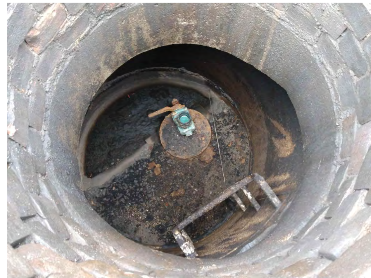
ACCESS POINT-17 INSPECTION PHOTO
