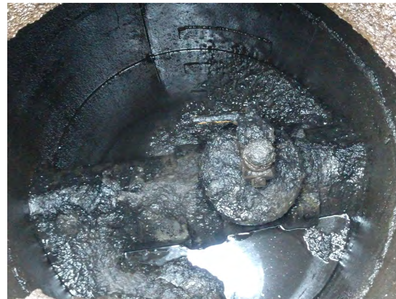
ACCESS POINT-14 INSPECTION PHOTO
