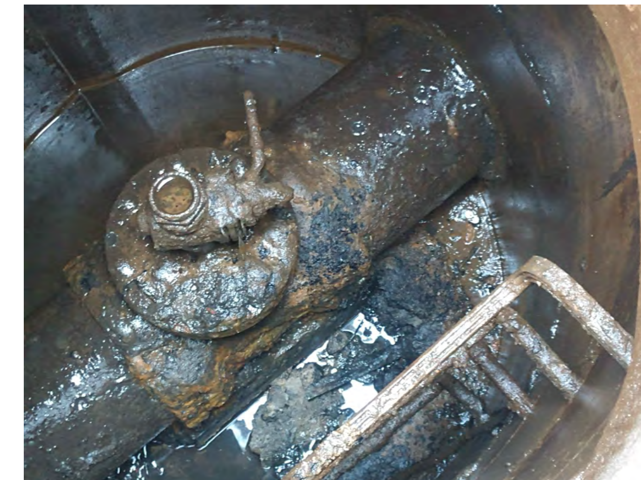
ACCESS POINT-12 INSPECTION PHOTO
