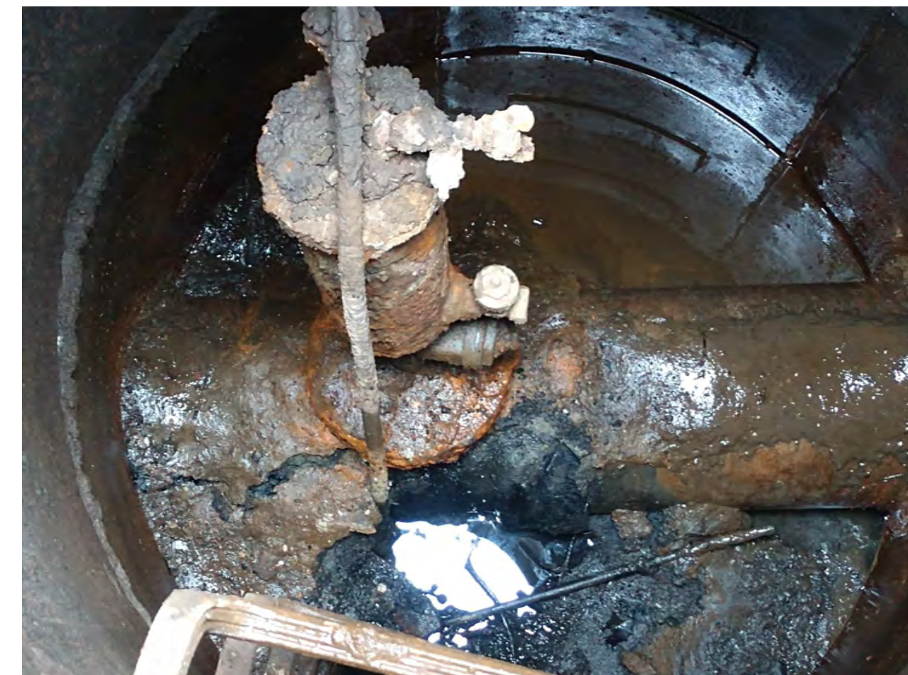
ACCESS POINT-13 INSPECTION PHOTO
